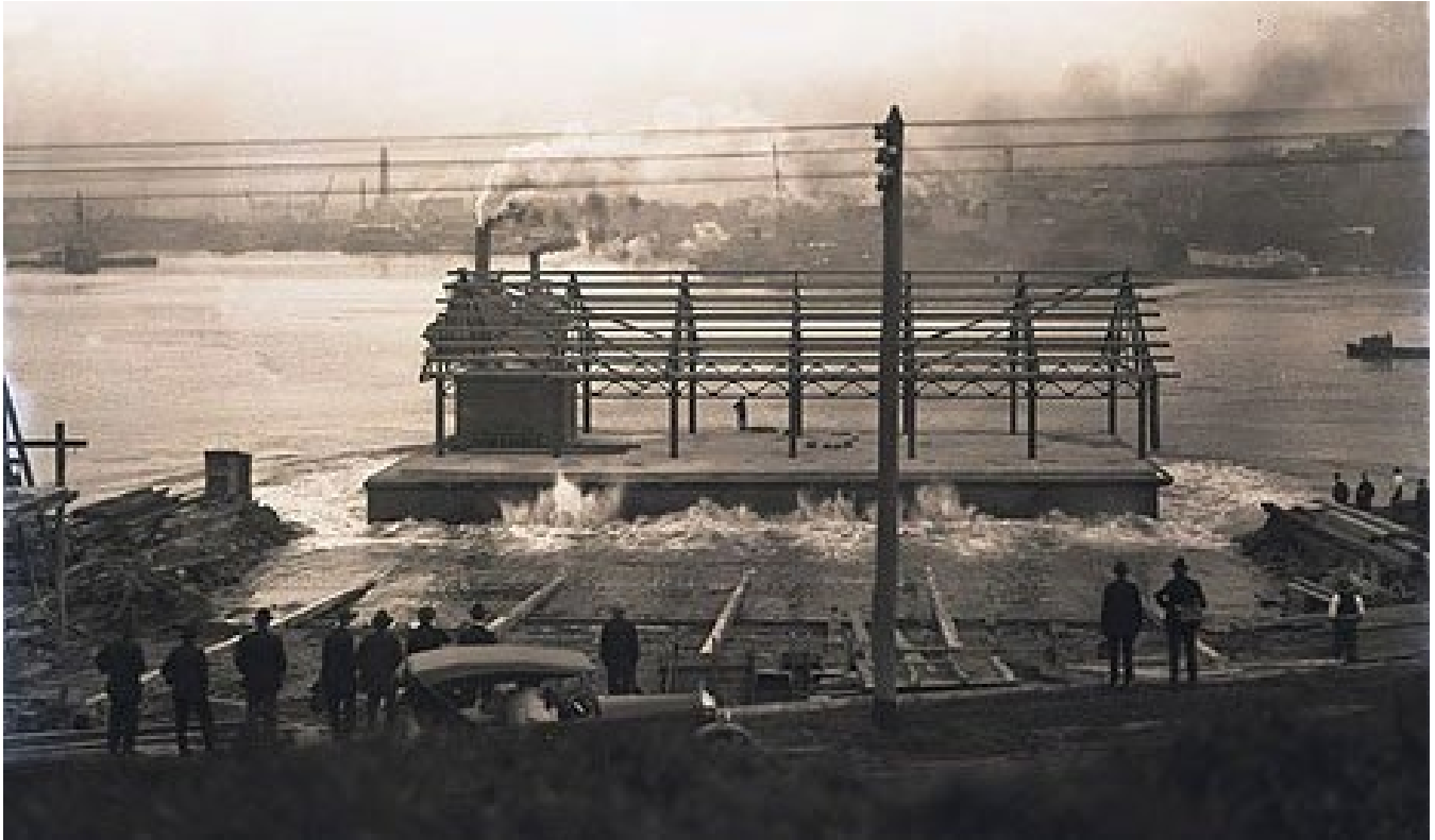
Floating wharf launch in Blackwattle Bay, 11 August 1924, Wikimedia Commons, Oxyman
