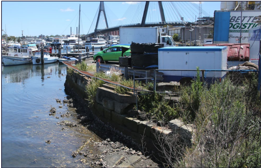
Photograph 3: Detail of sandstone seawall near former wharves of A & E Ellis (see Figure 9).
