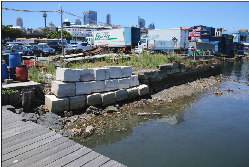
Photograph 4: Recent (2020) addition of sandstone blocks to shore up embankment at northern end of sandstone wall opposite A & E Ellis's former wharf. Compare to Photograph 5 taken in 2019 showing collapsing timber shoring.
