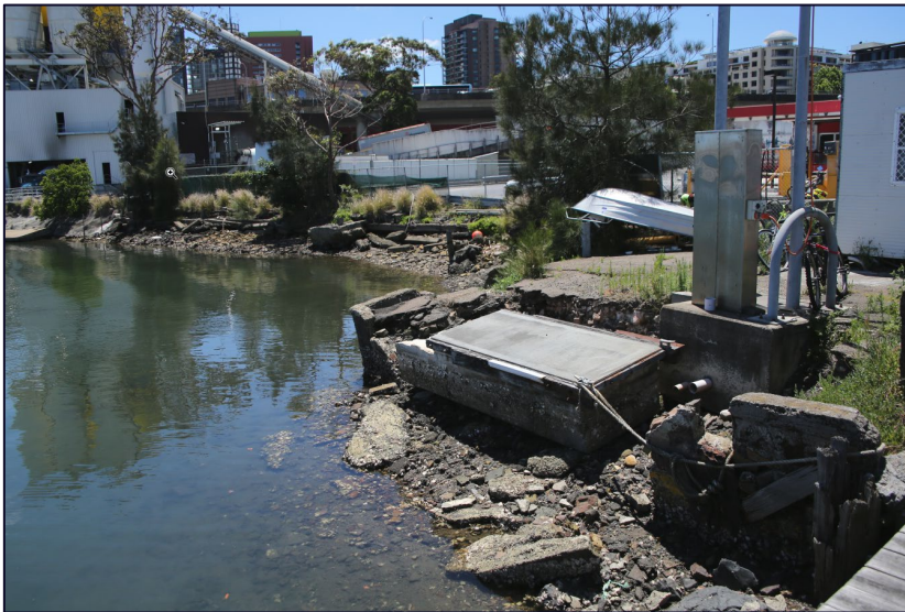
Photograph 6: 'Seawall' on northern side of jetty near former F Buckle & Sons site showing former piles and large horizontal timbers extending towards Hymix cement works site
