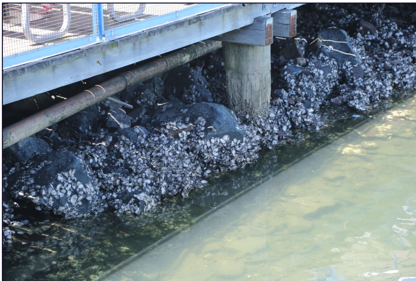
Photograph 12: The Sydney Fish Market boardwalk sits above sheathed and unsheathed timber pylons and layer of rock rubble
