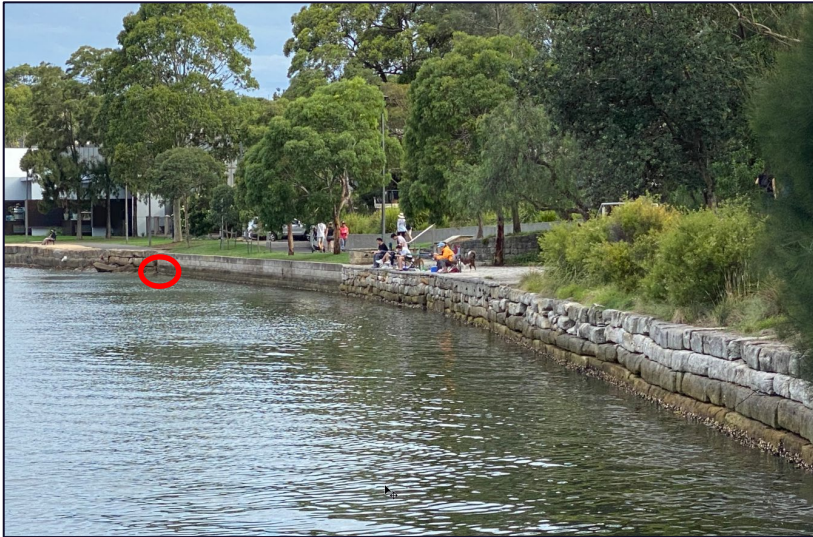
Photograph 22: Seawalls adjacent to the termination of Cook Street, Glebe. The sandstone blocks are either side of the concrete seawall which spans the termination of Cook Street. The location of the stone foundations of a wharf are circled in red. View to south-west.
