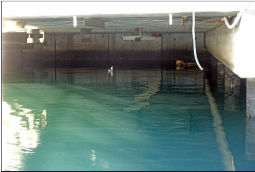
Photograph 16: Underside of the reinforced concrete deck of the wharf east of the coal loader showing seawall that runs the length of the site about 20m from Bridge Road.
