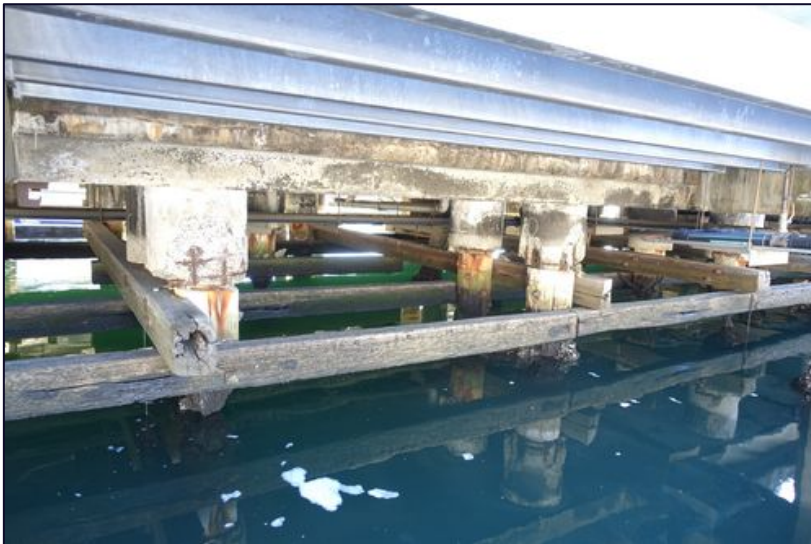
Photograph 17: Blackwattle Bay Marina B2 showing timber pylons and bracing beams prior to demolition in 2020.
