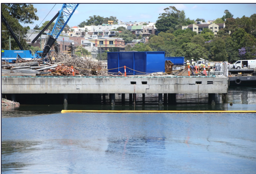
Photograph 15: Reinforced concrete deck of the wharf east of the coal loader showing seawall that runs the length of the site about 20m from Bridge Road.
