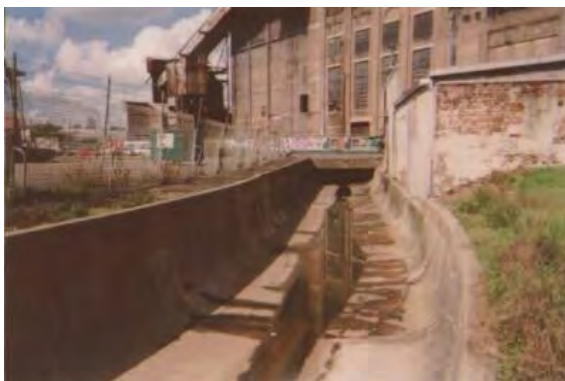
Figure 4.3.3.6: View of the stormwater channel north of Robert Street looking south toward the White Bay Power Station. (Heritage Office database. Date unknown but likely around 2001).
