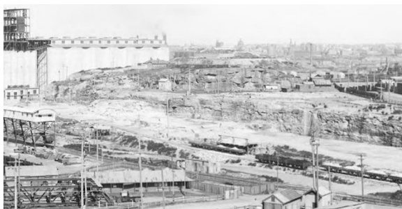
Figure 6.5.1: Extract of larger image undated. C1920. Photograph toward the first silo complex during construction c1920 including remnant sandstone cutting at that time. 20
