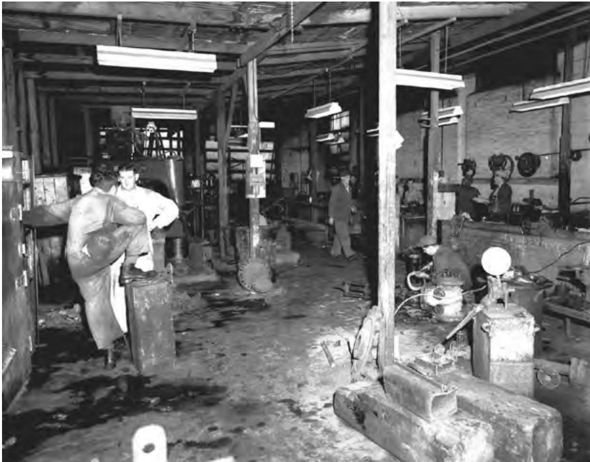
Figure 6.9.1: Working conditions in much of the power station was hot, dirty and noisy. This photo is dated 1959. 27
