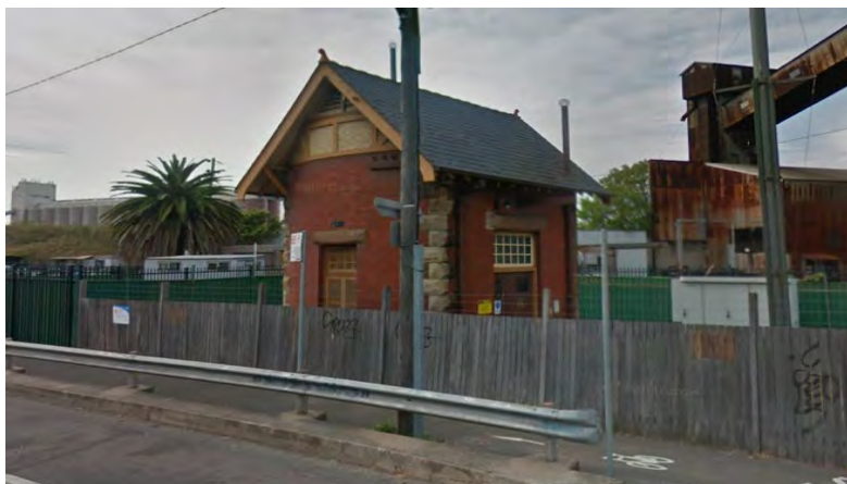
Figure 4.3.2.2: View of the Sewage Pumping Station 7 from Robert Street (Google Street View)
