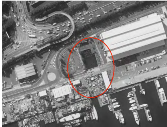
Figure 4.4.1.1: Aerial View of showing the location of the White Bay Power Station Outlet Canal. (Base plan: SIX Maps).
