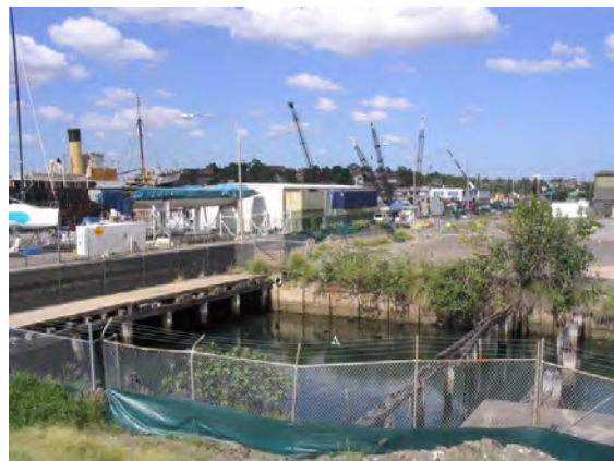
Figure 4.4.1.3: Photograph of the outlet canal opening near Rozelle Bay (Design 5, 2018)
