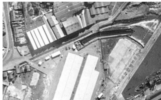
Figure 4.3.4.4: 1943 Aerial showing the open water coolant canal north of the northern penstock. (SIX Maps)
