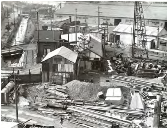
Figure 6.8.2: A number of small light framed buildings located around the site and power station.
