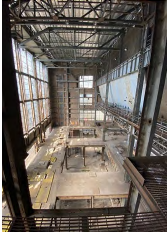
Figure 4.3.1.5: Boiler House looking south
