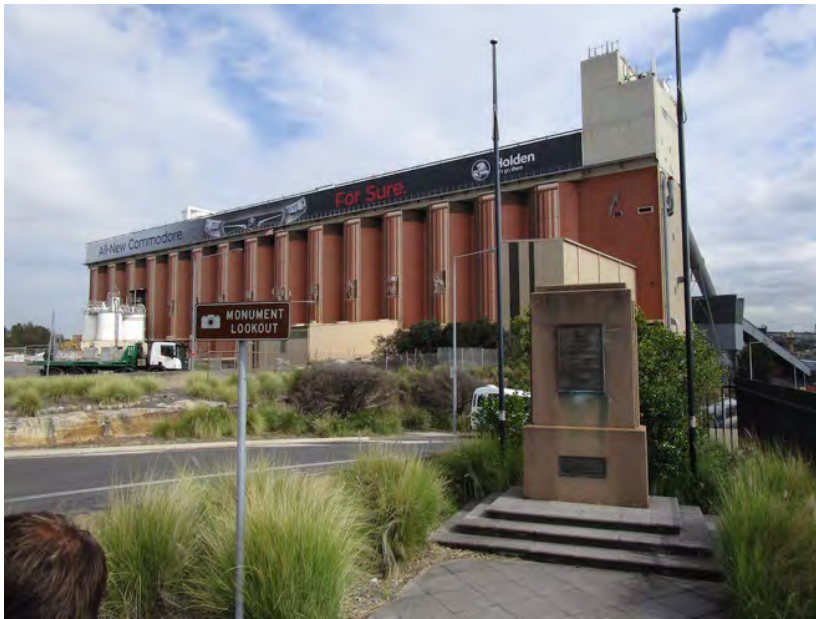
Figure 6.12.1: The monument commemorating the first landing of the United States armed forces at Glebe Island and the subsequent role of the Port authorities in moving personnel and supplies as part of the War effort
