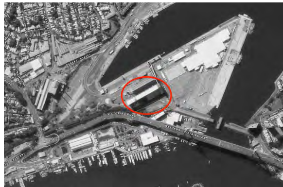
Figure 4.4.2.1: Aerial View of showing the location of the Glebe Island Wheat Silos. (Base plan: SIX Maps).
