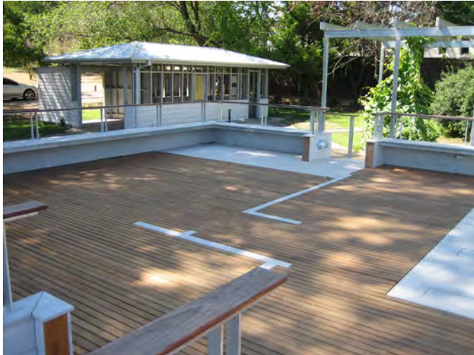
Figure 8.4.1: Interpretation of former Married Quarters at the Duntroon Royal Military College in Canberra. The former Married Quarters was interpreted as an outdoor deck with rooms and spaces outlined in the timber boarding. A signboard explains the significance of the building. The deck is used for outdoor gatherings and events within the college.
