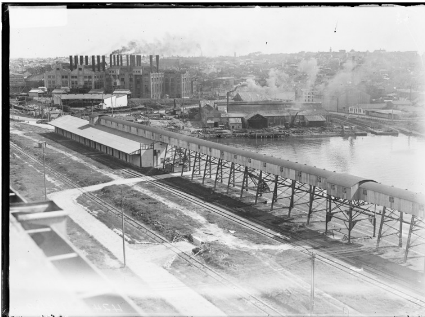
Figure 3.1.3.5: View from Glebe Island (likely from grain silos) toward White Bay. 9
