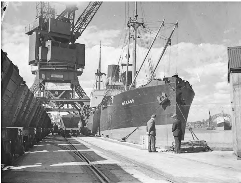
Figure 6.7.2: Coal being loaded onto shipping at White Bay. 26
