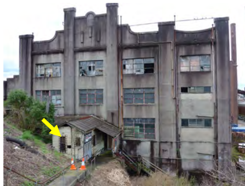
Figure 6.8.5: Image shows the former canteen attached to the south elevation of the Admin building that was demolished in 2011 due to hazardous materials and poor condition.
