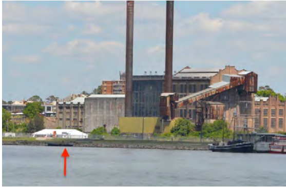
Figure 4.3.4.1: View toward White Bay Power Station from White Bay. The arrow indicates the location of the inlet canal.
