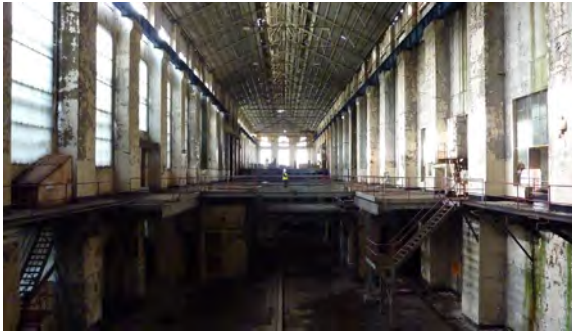
Figure 4.3.1.3: Turbine Hall looking north
