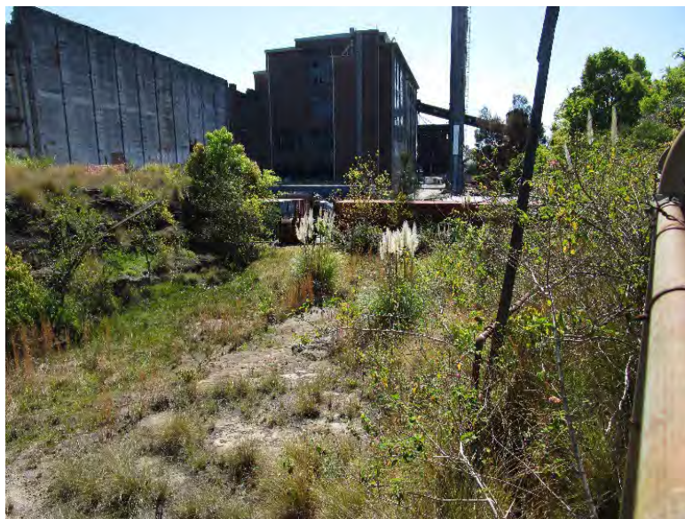
Figure 7.2.5: Rail connections to the Power Station.
