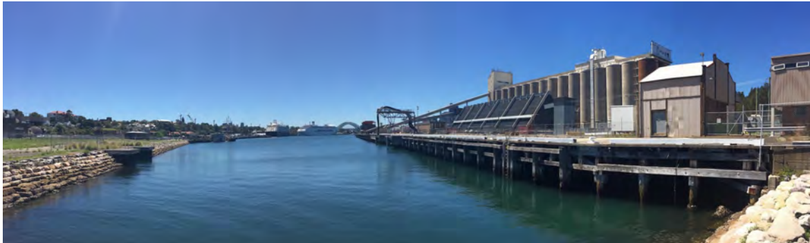
Figure 5.1.4: View looking from the head of White Bay to the north toward the Glebe Island and the Harbour Bridge.
