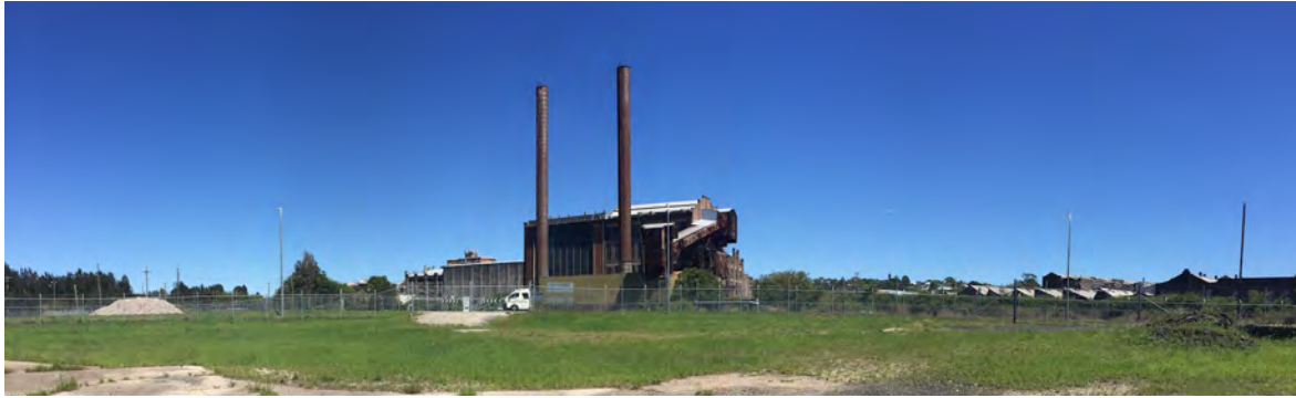
Figure 5.1.3: View looking toward the White Bay Power Station from the head of White Bay.
