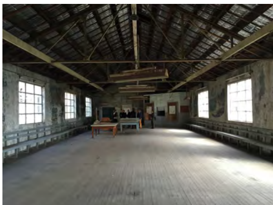
Figure 6.9.1.2: Existing photograph of the Entertainment Hall of the White Bay Power Station
