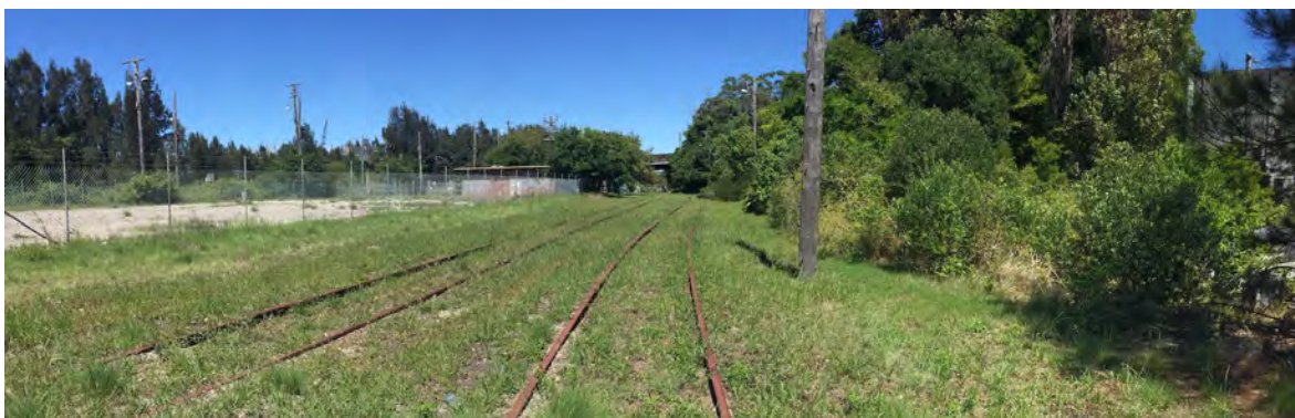
Figure 5.1.2: View along the rail corridor looking south.
