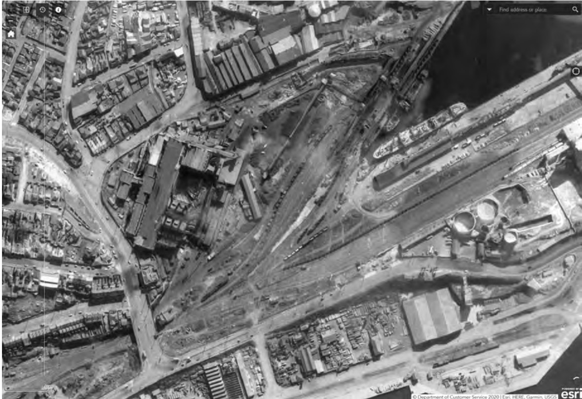
Figure 6.6.2: Aerial of White Bay and Glebe Island in 1955 showing the importance and interdependency of rail corridors for goods export, White Bay Power Station, grain silos and connections to Darling Harbour 24 .
