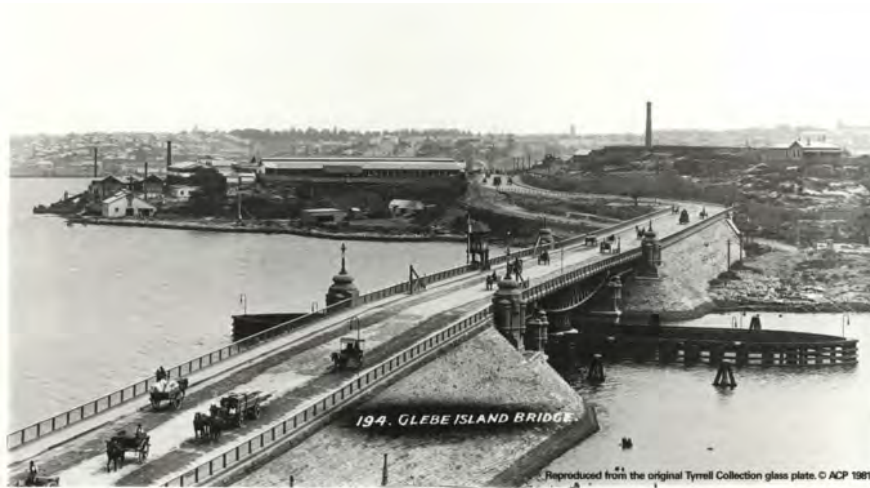
Figure 3.1.3.1: Glebe Island Bridge in 1910 – image cropped. 5
