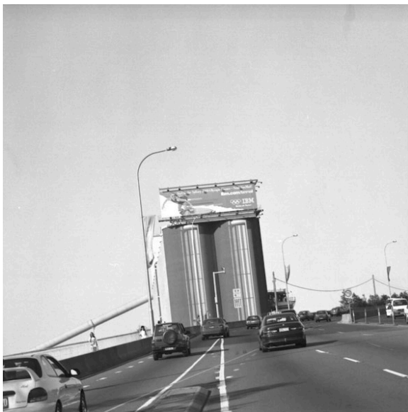
Figure 4.4.2.3: View of the Silos from west approach in September 2000. 14
