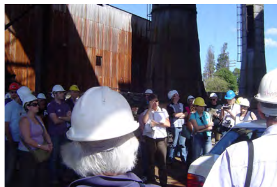
Figure 9.4.4: Tours of the White Bay Power Station have occurred in the past on public open days and specialist tours for professionals.
