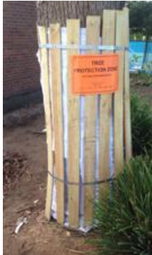
Figure 3: Trunk protection
