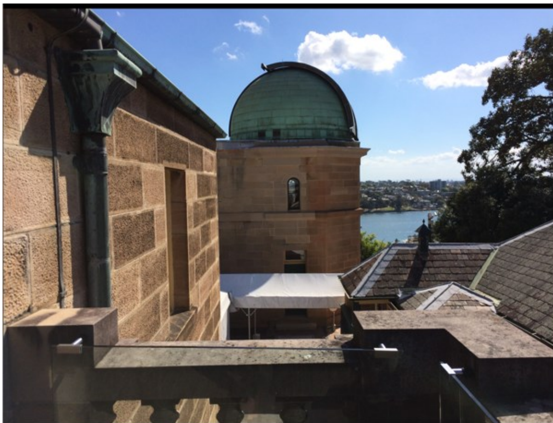
Photo 2 – View from Sydney Observatory looking west towards the north dome (note the height above sea level of the horizon in the background). The observing deck is located just to the left of the north dome and is concealed by the sandstone building in the foreground.
