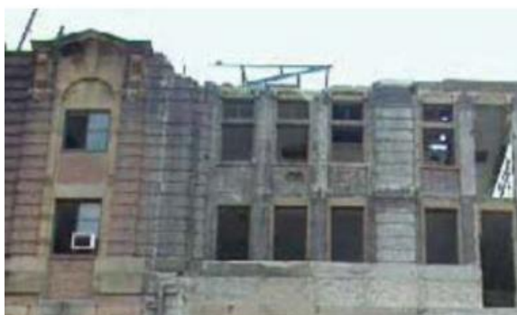
Figure 7 – 1993 Severely dilapidated eastern façade.
