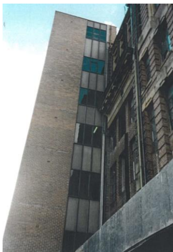
Figure 5 – 1960s Annex to eastern façade.
