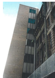
1960's annex to Eastern elevation
