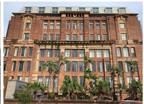
/ Current rebuilt Eastern elevation
