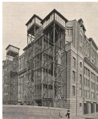
/ Lift attachments to Eastern elevation
