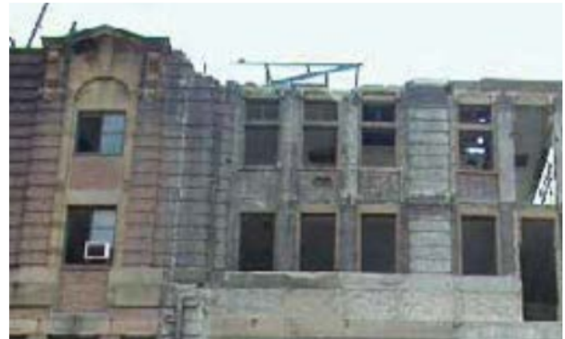
Eastern Facade in dilapidated condition - 1993
