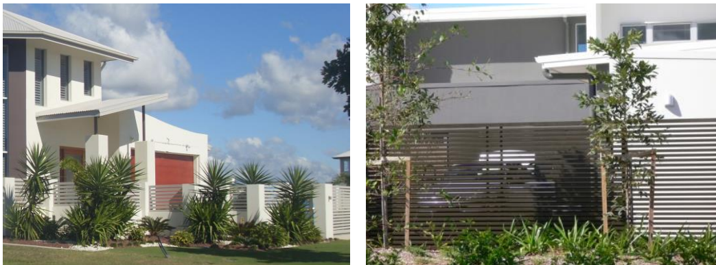
Figure 2.2.24.4 Examples of Translucent Fencing on a Secondary Boundary of a Corner Site
