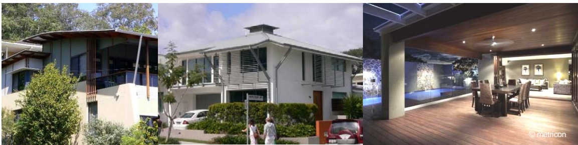
Figure 3.1.3.5 Examples of desirable climatically responsible design, wide eaves, deep shaded Private Open Space areas.
