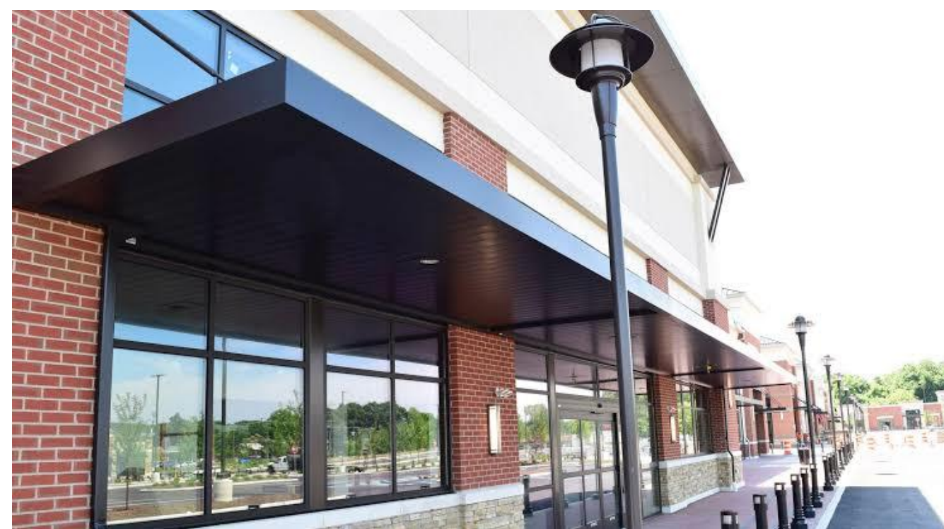
METAL AWNING OVER SHOP FRONT DOORS
