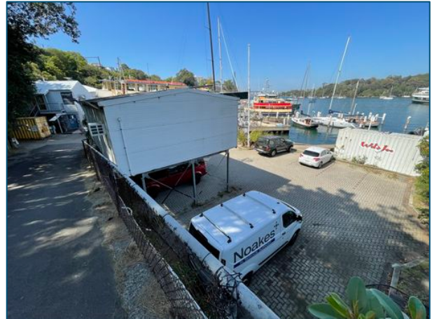
Photograph 10: Vehicular entrance and paved area at northern end of site. Brick paving is onto fill. View to south-south-west.
