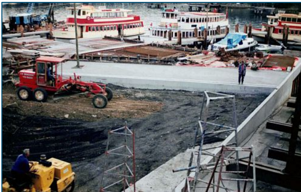
Photograph 7: Spreading of fill behind concrete retaining walls
