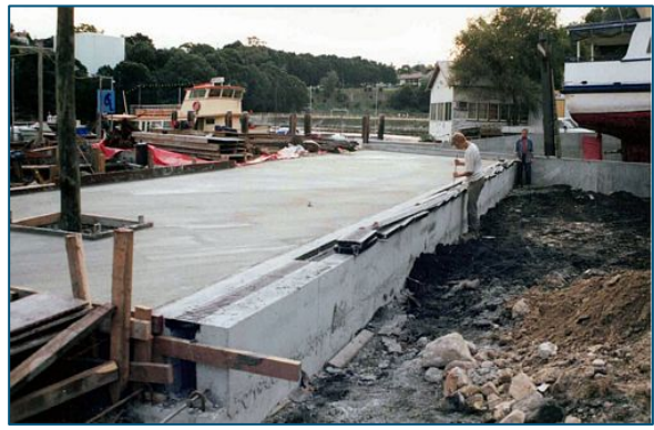
Photograph 6: Concrete slab wharf hardstand
