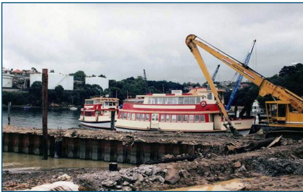
Photograph 5: Introduced fill for new wharf
