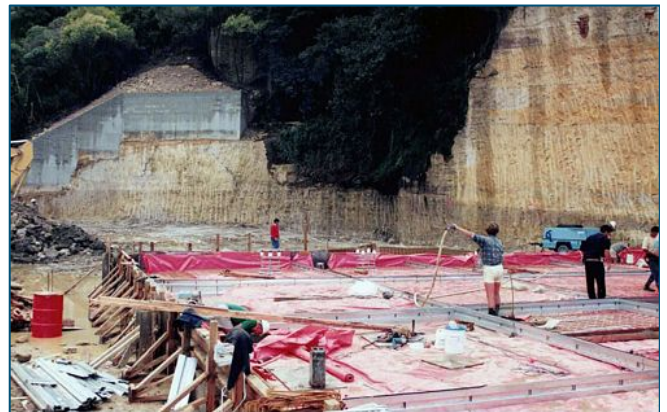
Photograph 2: View to north-east showing excavated rock wall and laying of concrete slab for large, open, work sheds
