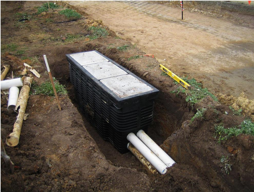
Figure 6-3 | "9 Pit" with multiple P100 conduits being installed
