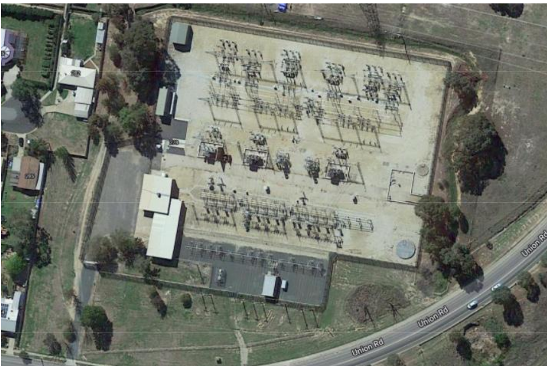
Figure 5-2 | Existing Union Road substation (Source: Essential Energy DAPR – Rosetta Data Portal)
