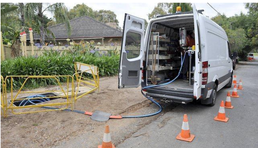
Figure 6-4 | Splicing Van Accessing a roadside pit
