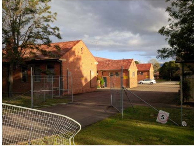
9 Albert Street: Single Storey buildings and yard area
