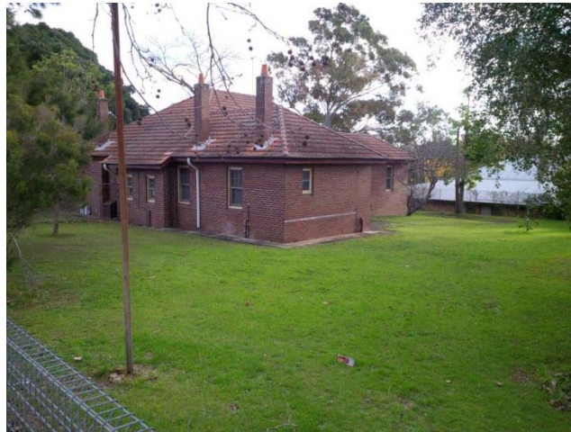
2D Fennell Street: Cottage signed as Eating Disorders Day Hospital Program. Lilian Wells Nursing Home roof line to the West of the building
