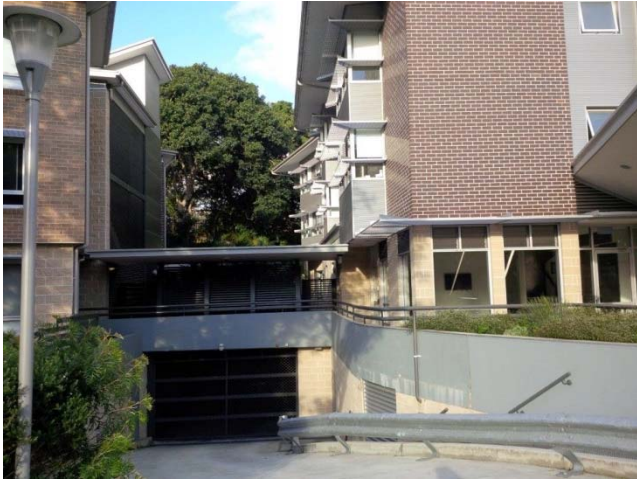
2B Fleet Street, new residential development with basement sublevel apparent (assisted/community housing)
