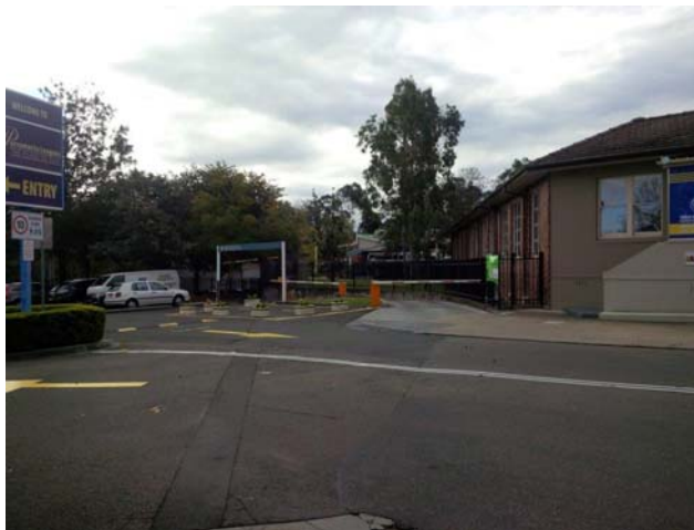
1 Fennell Street: Southern extent of the Northcott Society development including entry to the basement level car park from the Eels Club car park.
