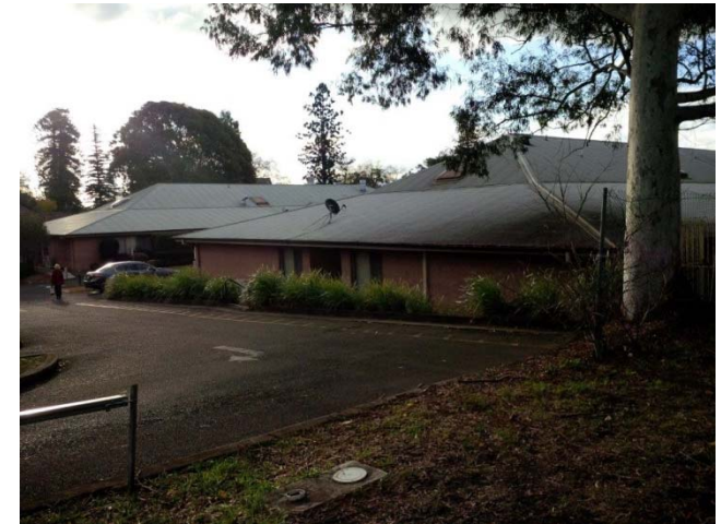
2A Fennell Street: Lilian Wells Nursing Home Buildings looking Toward the north-west.
