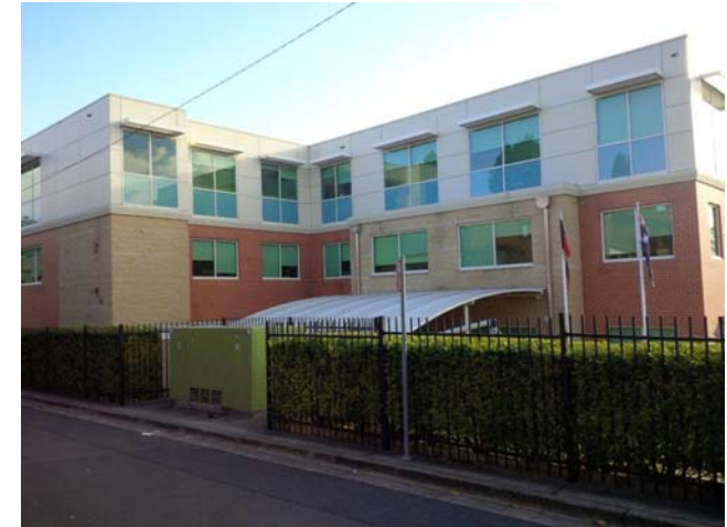
1 Fennell Street: East portion of the Northcott Society from Laneway to the east, including electrical transformer.
