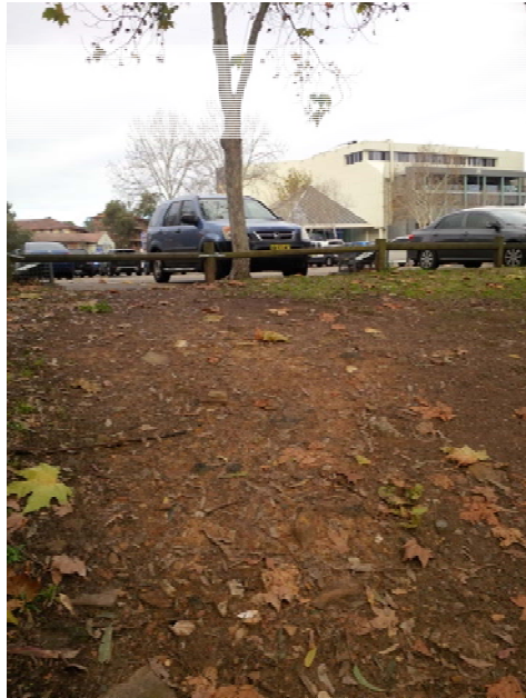
Exposed Fill Embankment at West extent of Eels Club carpark with the Leagues club building in the Background.
