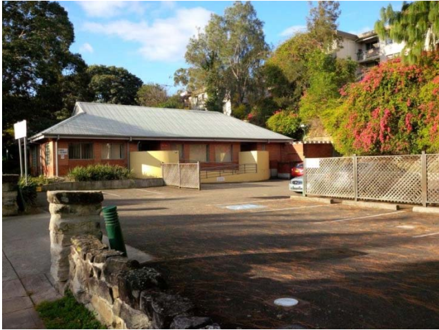
Fleet St OUT WSLHD Building and carpark. Exposed Sandstone face at rear of the site.
