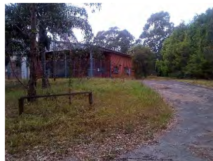
Vacant Lands – Building 4, stores. 1990s construction on Filled platform
