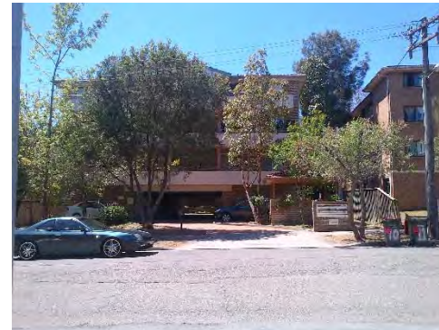
New St Residences Site portion
