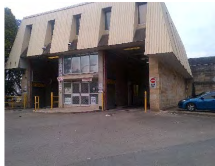
Linen Service – Entrance Building (Building 2)
