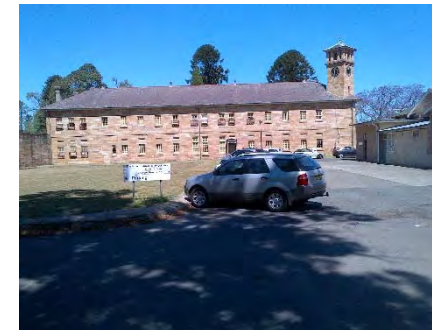
Building 90 looking toward the west.
