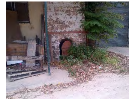
Vacant Lands – Base of chimney Stack in Building 17 (Pol AG)
