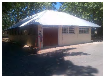
Building 94 looking south.
