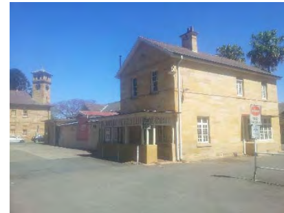
East Campus: Building 89, looking toward west with Building 90 in background.
