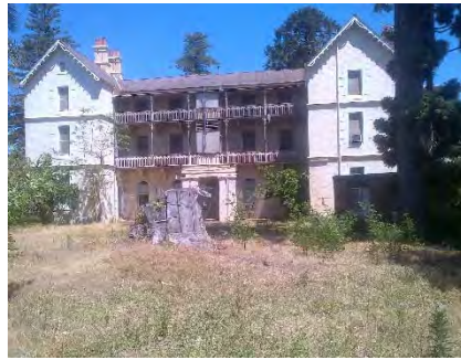
Norma Parker – main building (105) looking south-west
