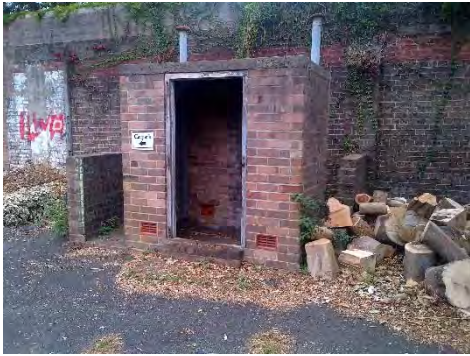
Kamballa – Inferred former dangerous goods storage facility (Building 114).
