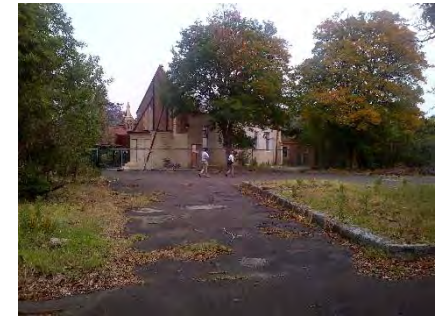
Norma Parker – Main Yard with fire damaged building 107 (Pol AY). Looking south-west from Building 109.
