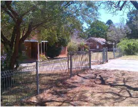
East Campus - Two CHIP Cottages at east of site (Buildings 59 and 42)
