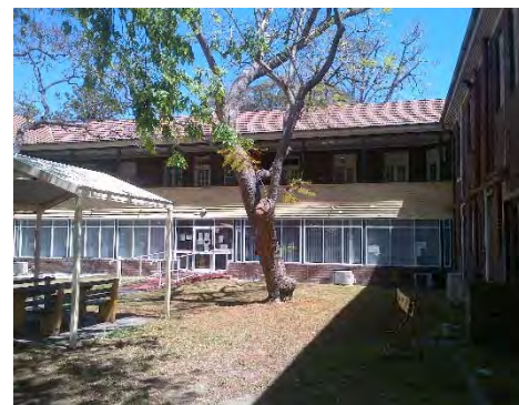
East Campus - Internal Courtyard Building 58
