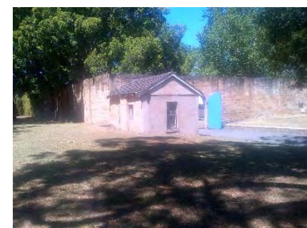
Building 88 with artisans compound wall at rear (south).
