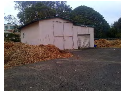
Kamballa – Building 113, maintenance shed adjacent to East site fence, surrounded by mulch stockpiles
