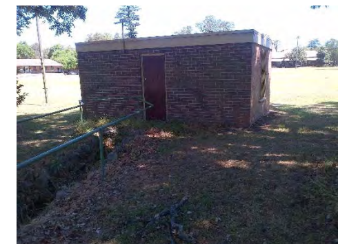
East Campus - Building 56 and drainage channel to east
