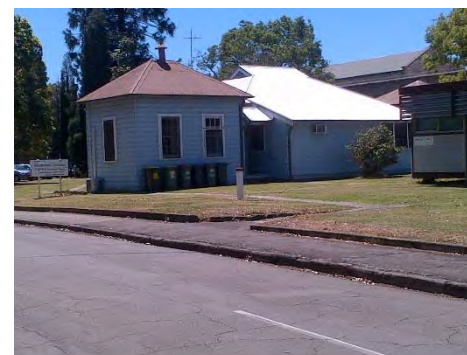
East Campus - Building 34 looking to north east
