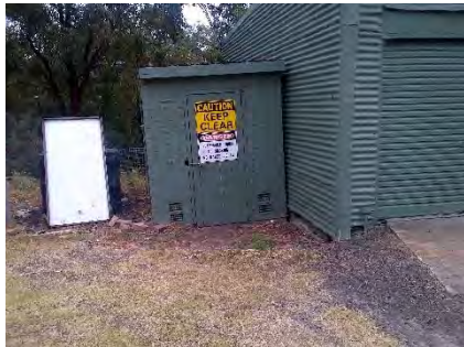
Vacant Lands – Hazardous Goods store (Building 30)
