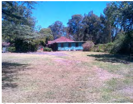
East Campus – Building 51, looking south. Former building foundations apparent in the foreground
