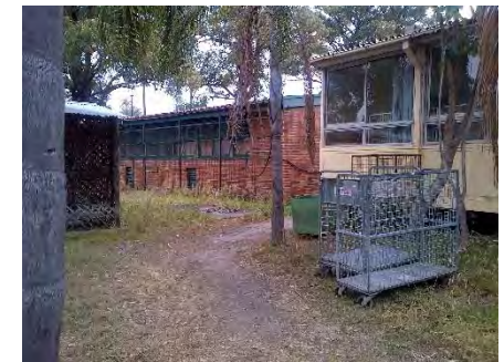
Vacant Lands – Building 15 on right, 13 at the centre and 13 (shade structure on the left)
