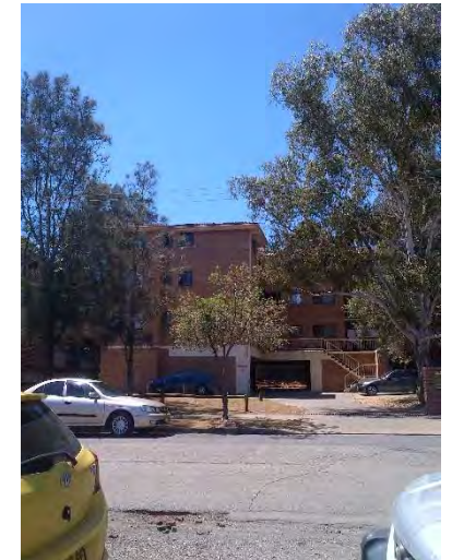
New St Residences Site portion
