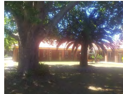
East Campus: Substation facilities Building 73 courtyard (above) and fibro clad Shed at rear of building (right).
