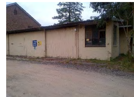
Vacant Lands – Former maintenance workshop portion of Building 17.
