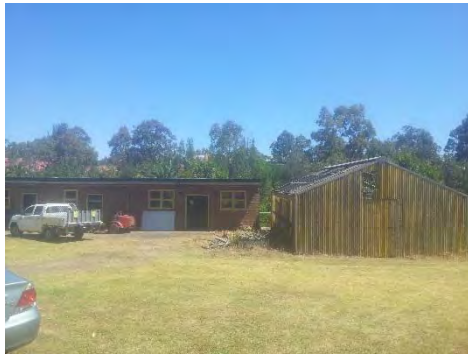
East Campus – Gardener's Store and former greenhouse to north. Facing West (Building 68)
