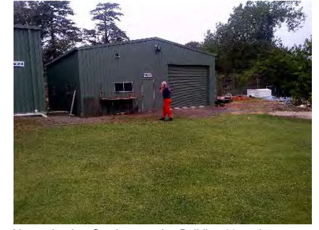
Vacant lands – Southern portion Building 28, maintenance Workshop with filled area to right (west).
