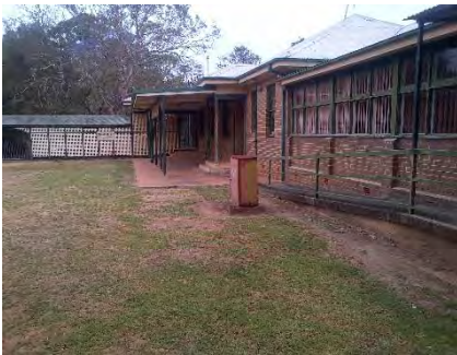
Kamballa – Building 117 looking south-west
