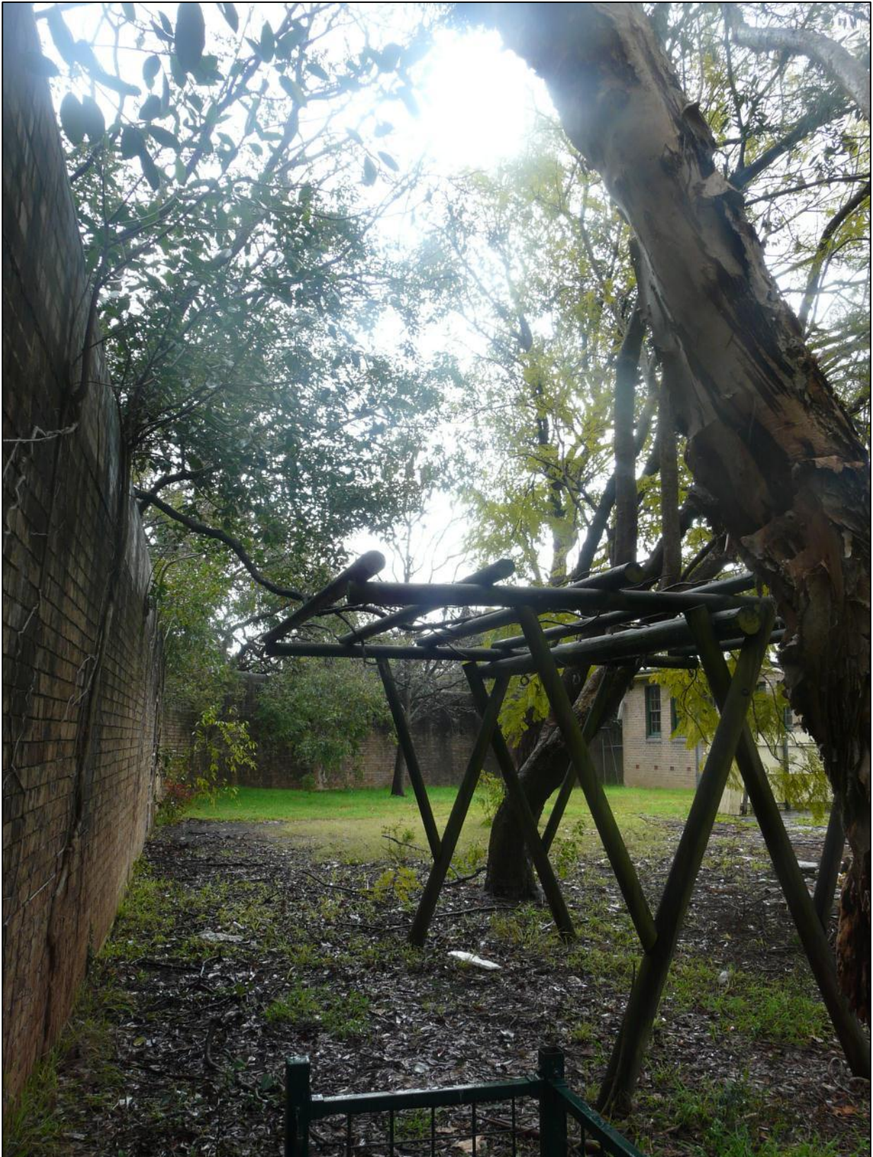
Figure 6: Wall to be retained between the GHFF camp and adjacent uses (view from eastern side)
