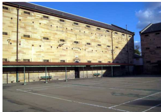
55 Cell Block 5 (1880s) with the exercise yard in the foreground.
