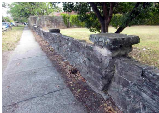
73 The sandstone kerbs on Fleet Street.
