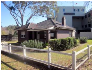
The Ross Street Gatehouse
