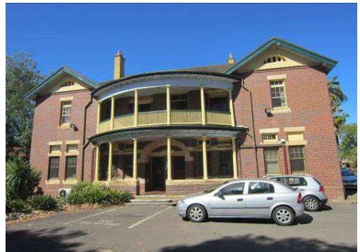
33 The former Administration Block of the Parramatta Hospital for the Insane.
