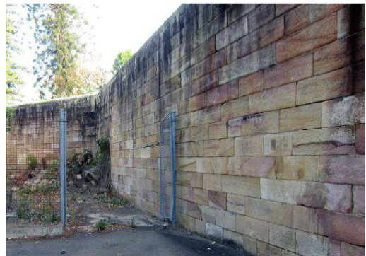
21 The sandstone compound wall of the former Cell Block Extension.
