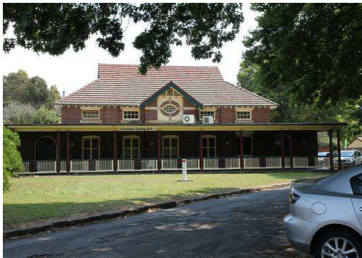
24 'The Staff Dining Room designed by WL Vernon who was the NSW Government Architect.
