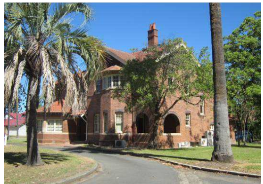
35 Jacaranda House—a former nurses home constructed by WL Vernon.
