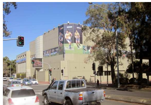
77 The multi-storey Parramatta leagues Club building on O'Connell Street.
