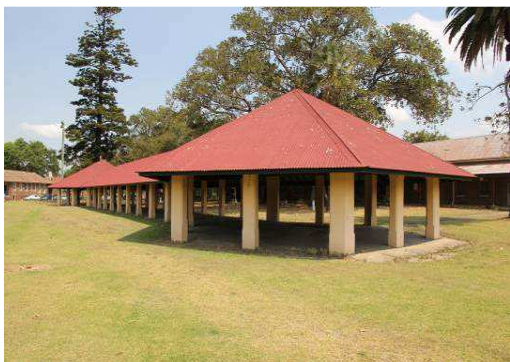
28 The former Male Shelter Shed and pavilion.
