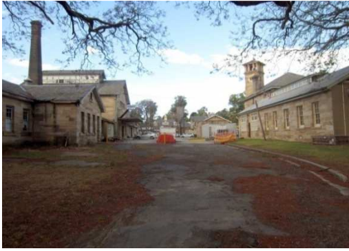
14 A view of the sandstone buildings of the former Female Factory and Lunatic Asylum.
