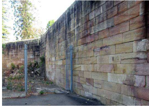
23 The sandstone compound wall of the former Cell Block Extension.
