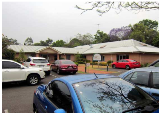
71 The Lilian Wells Nursing Home on Fennell Street across the road from the Northcott Centre.
