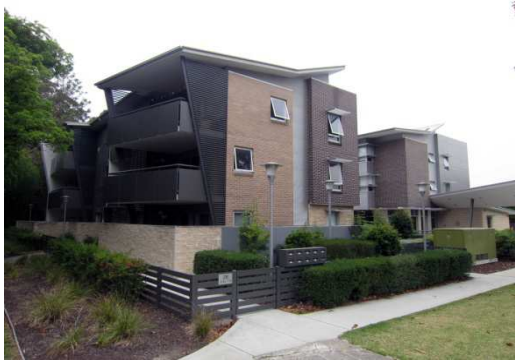
68 The newly constructed Hope Hostel (incorporating the Hope Apartments) on Fleet Street.
