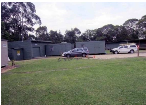
36 The SES sheds located at the northern end of the study area.
