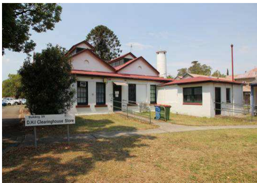
26 The former Kitchen Block and Store buildings. The chimney stack was truncated in the 1960s.
