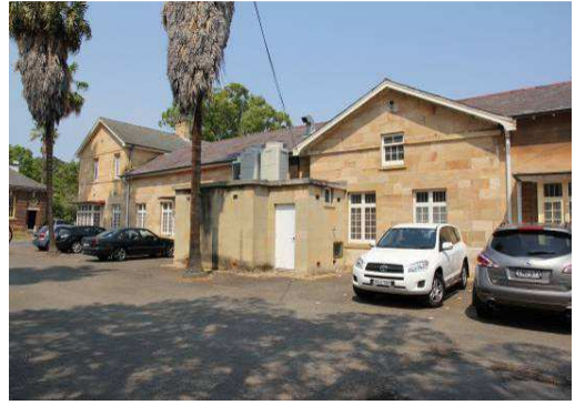
15 The northeast wing of the former Female Factory, which has undergone significant modification.
