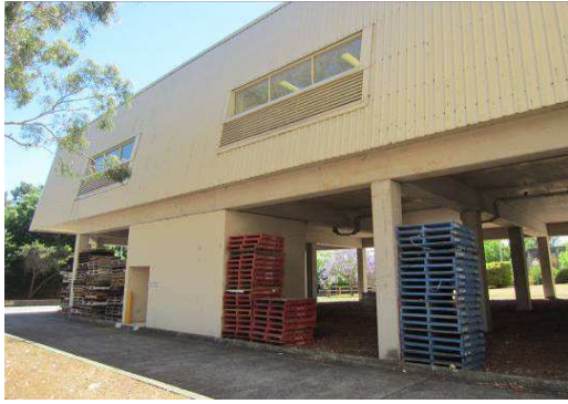
58 The main Linen Service building constructed within the former Parramatta Gaol Farm area.
