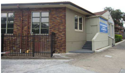
72 The Parramatta Leagues Club support building on Grose Street.
