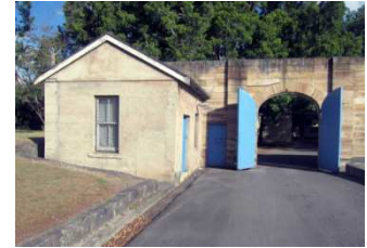
The former Dead House and entry to Cell Block Extension
