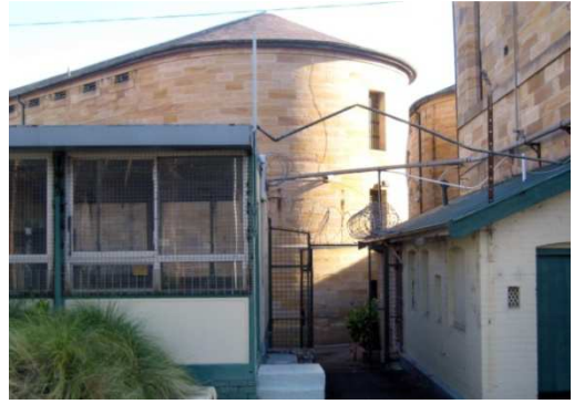
51 Cell Wing 3 at Parramatta Gaol. The 1990s demountable can be seen in the foreground.
