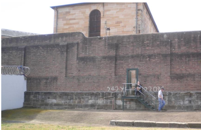
Figure 3.30: Eastern boundary wall of oval; the lower sandstone courses may have been the earliest rear boundary of the gaol complex. Note the lower level of the oval compared to the eastern half of the gaol. Photo taken 29/07/2014, by NP.
