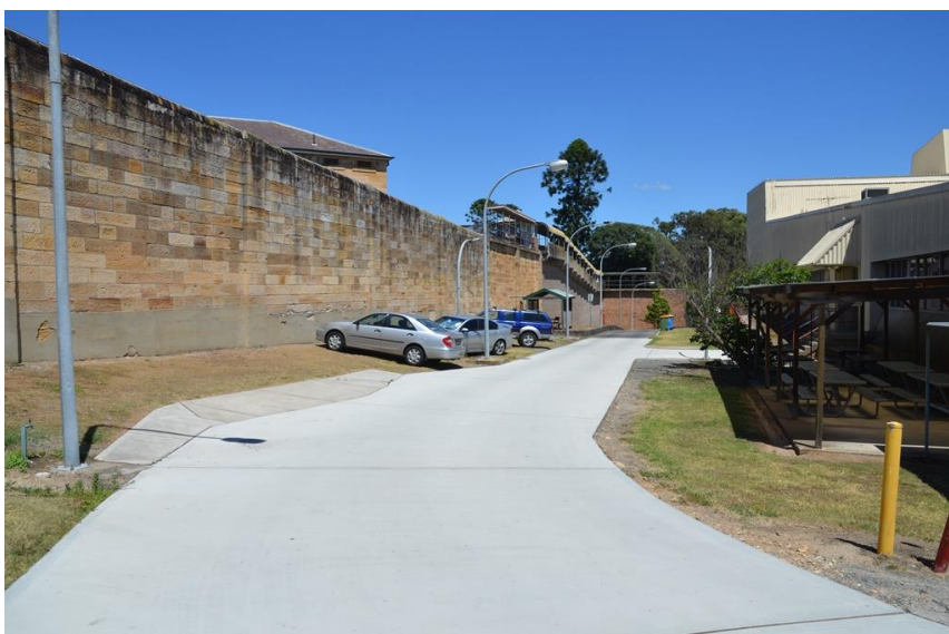
Figure 3.36: View to west along the southern boundary wall with the Gaol.
