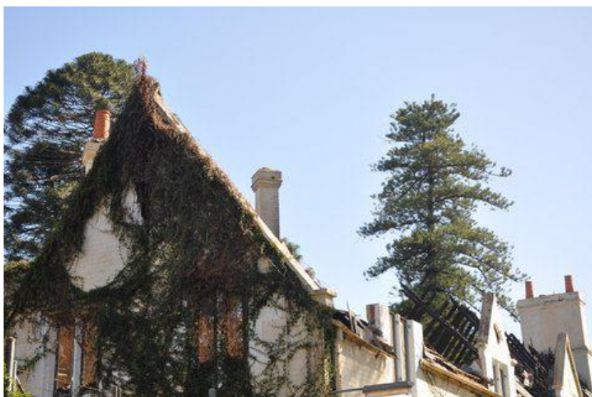
Figure 3.57: Photo showing damage to the roof from the 2012 fire, Greater Western Sydney Heritage Action Group Facebook page, Norma Parker Centre Fire December 2012 Album. Accessed on 31/07/2014.
