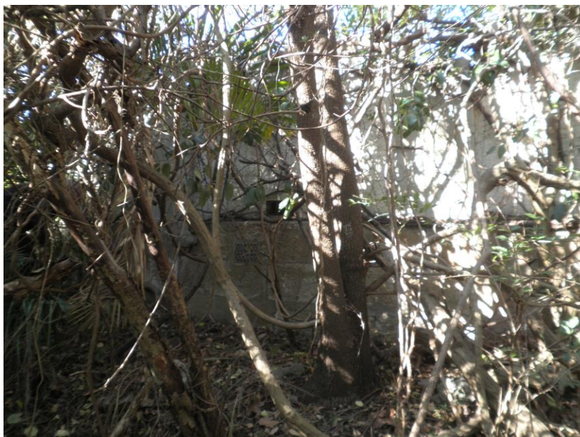
Figure 3.23: Rendered wall and sandstone retaining wall. Taken looking east, 29/07/2014, by NP.
