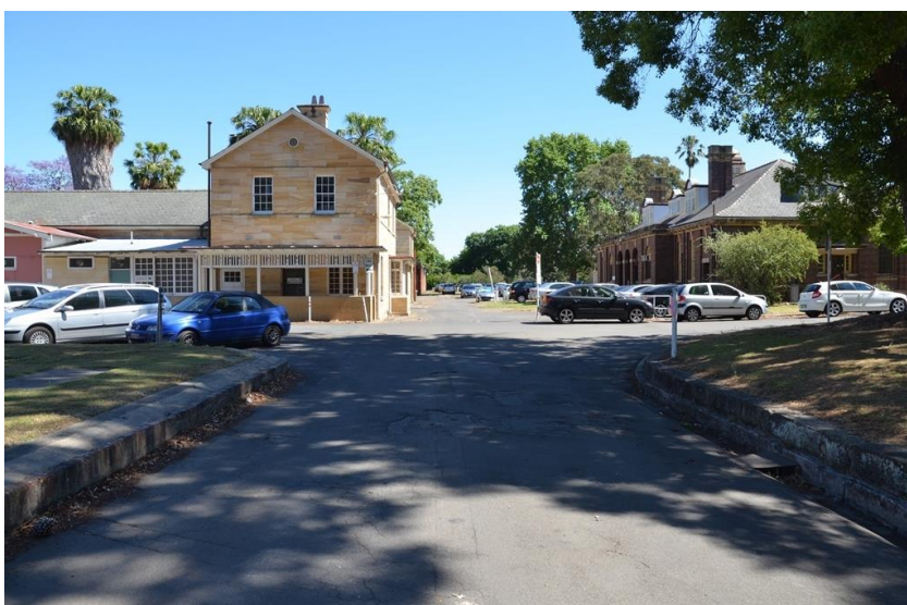
Figure 3.4: Looking north with the later Administration building on the right and original Factory buildings on left. The remains of the Factory wall and the moat or mill race should be in this area.
