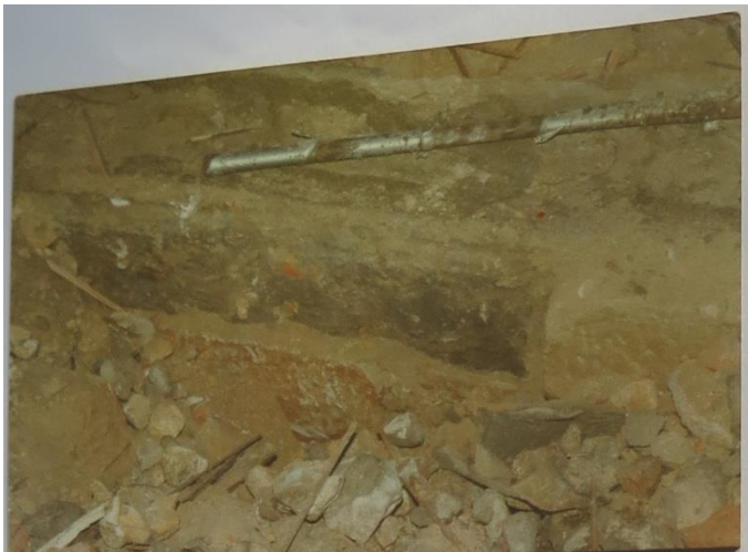
Figure 4.15: Footings of an early wall observed during building works under Ward No. 5 (now building 104) in October 1985. Photograph from Terry Smith Collection.
