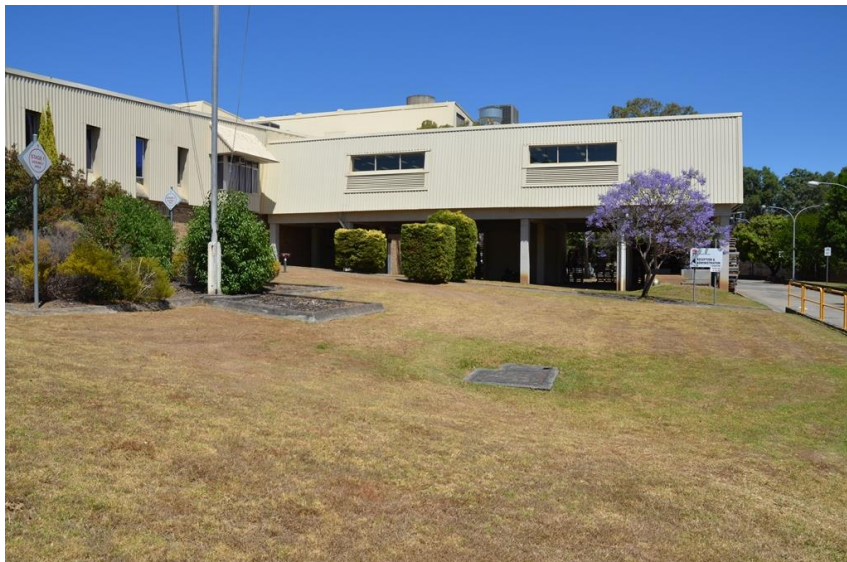
Figure 3.38: New building erected in 2005-06 on piers.
