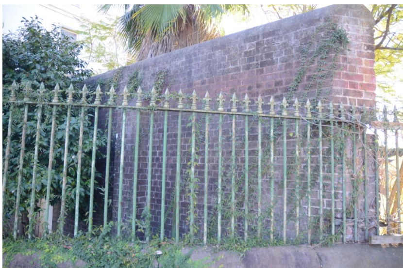
Figure 3.55: Intersection of the sandstone and iron palisade fence along Fleet Street, with a section of the internal brick fence. Looking west from Fleet Street, 29/07/2014, by TL.
