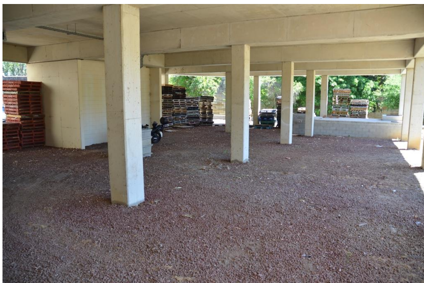
Figure 3.39: All pile areas were subject to archaeological testing in 2005-06 by AHMS.
