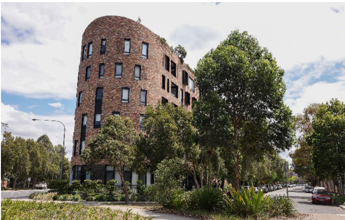
Figure 5. Residential flat building on Huntley Street, Alexandria
