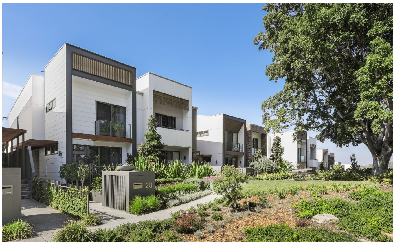
Figure 12. Dual occupancy housing in Ryde
