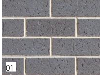
EXTERNAL BRICK WALLS FACE BRICK - PGH OLYMPUS
