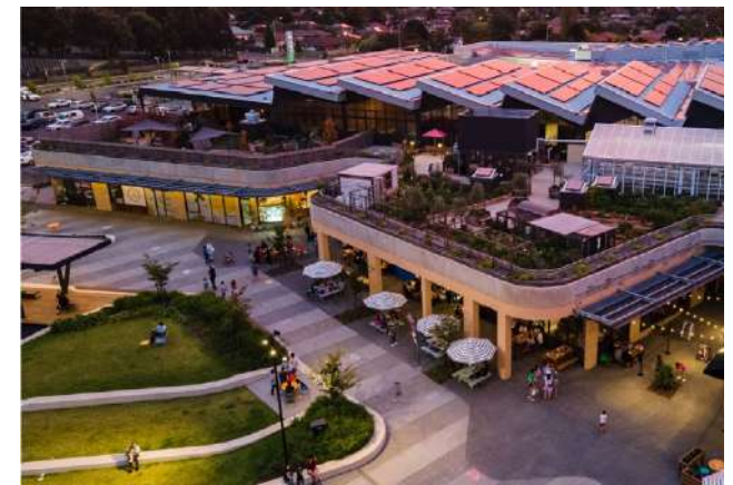
Co-location of retail, public space, residential, entertainment and an urban farm. Burwood Brickworks, Melbourne
