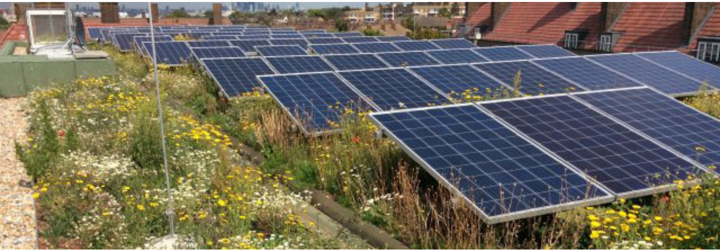
Figure 2.9 Biosolar roof combining solar panels with green roof (Source: Living Roofs)
