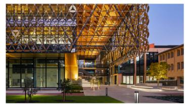
A veil façade with petals fixed at different angles to suit their orientation mitigates glare, heat, and filters sunlight.
