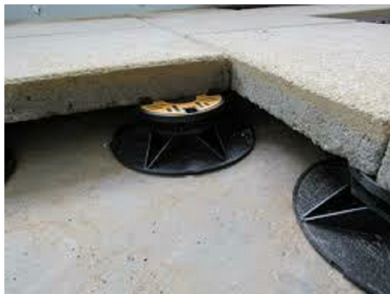
EXAMPLE OF POD AND PAVER SYSTEM
