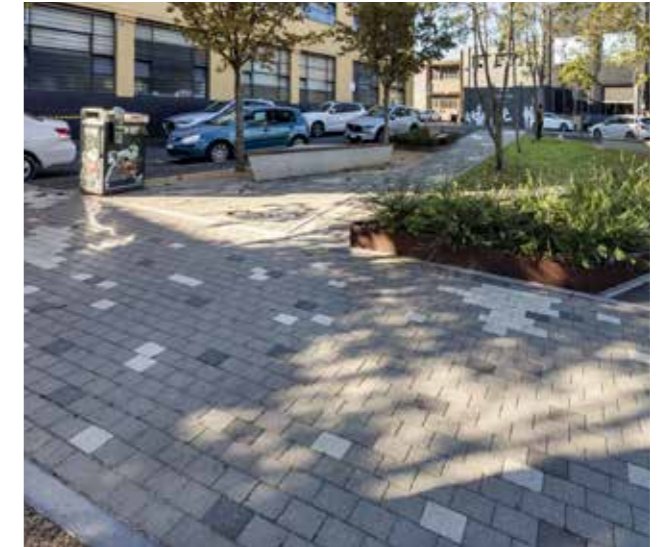
Porous paving: Permeable paving helps stormwater soak into the ground and street trees to thrive.
