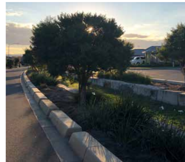
Raingardens: A central swale captures runoff and provides passive irrigation to central median trees and groundcover plants.
